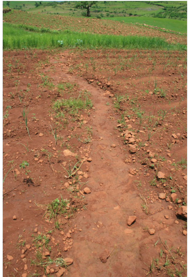
Fig. 21.3 Rill erosion at a farmer's field at Wonzima (Blue Nile basin). Rills occur particularly on long and steep slopes without soil conservation structures; here, the depth of the rill is controlled by the tillage pan, on which plough marks of the ard are visible (Photograph E. Monsieurs, August 2013)
