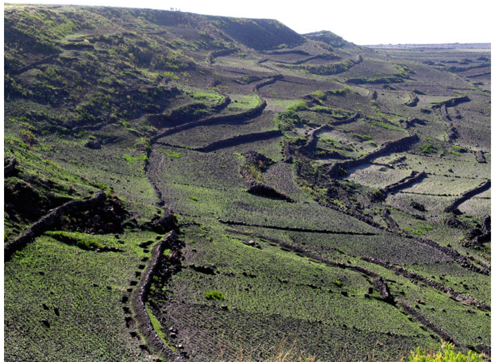
Fig. 21.8 Catchment rehabilitation in the sub-humid May Zeg-zeg catchment (Tigray); trenches behind the stone bunds enhance infiltration and decrease catchment runoff response (Photograph K. Herweg, May 2005)
